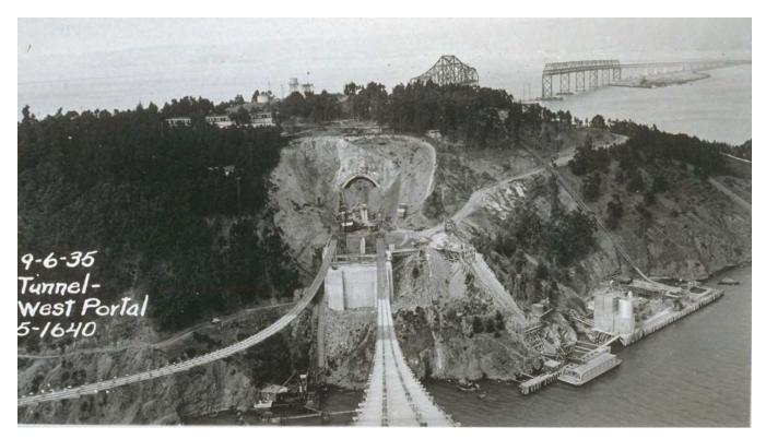
Figure 79. West Portal of the Yerba Buena Tunnel during construction of the San Francisco–Oakland Bay Bridge, as seen from the first tower of the western span; notice eastern span in background (Bancroft Library Collection).
