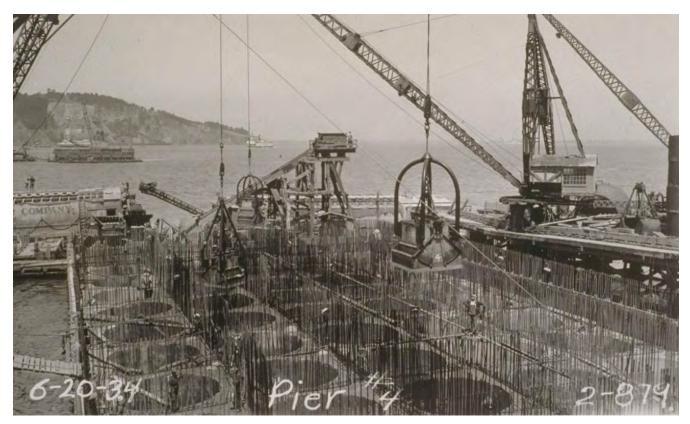
**Figure 78.** Excavation of central anchorage caissons on the western span of the San Francisco–Oakland Bay Bridge (Bancroft Library Collection).
