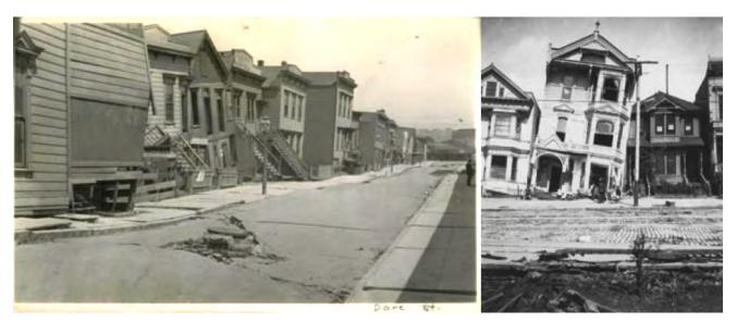
**Figure 50.** Liquefaction-related damage in San Francisco due to the 1906 earthquake. Photograph on left shows Dore Street (from Bancroft Library) and photograph on right shows an area near Howard & 17<sup>th</sup> Streets (G.K. Gilbert, USGS photo).
