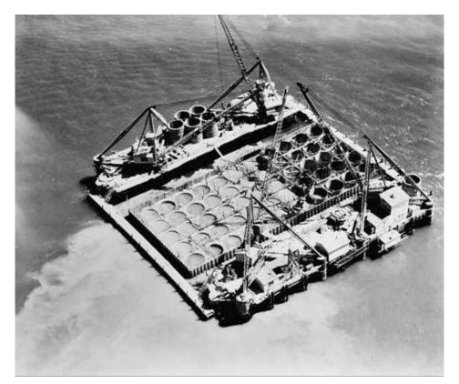
**Figure 77.** Construction of the caisson system for the central anchorage on the western span of the San Francisco–Oakland Bay Bridge (Bancroft Library Collection).
