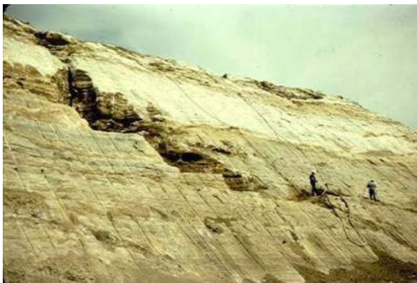
Figure 3-12 Solution features exposed during earthworks for the Clarence Cannon Dam, central Missouri. Courtesy of J. Higgins, Colorado School of Mines.
