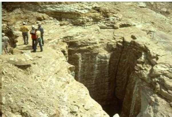
Figure 3-12 Solution features exposed during earthworks for the Clarence Cannon Dam, central Missouri. Courtesy of J. Higgins, Colorado School of Mines.
