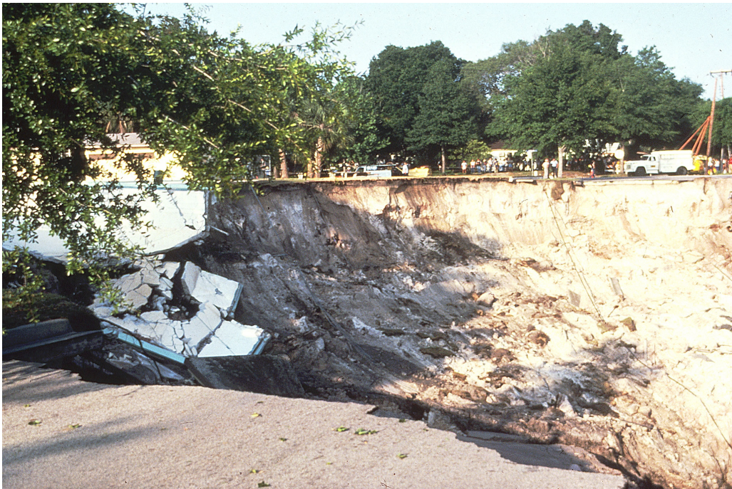
Figure 3-9 Surface collapse of cohesive soils above a sinkhole in Winter Park, Florida. Note vehicles in the foreground for scale. From https://www.usgs.gov/media/images/winter-park-florida-sinkhole-1981-12
