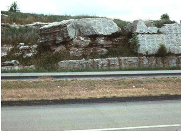
Figure 3-10 Pinnacled bedrock. Top: highly developed, exposed on a construction site in China. From Waltham and Fookes (2005); Bottom: moderately developed, exposed in a 6 metre roadcut. Courtesy of J. Higgins, Colorado School of Mines.
