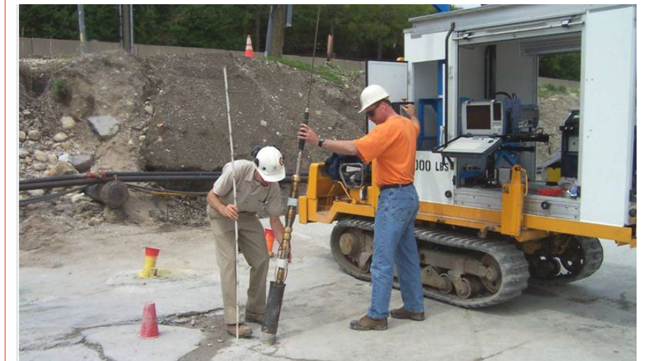
Logging core holes [TOP] and using an optical televiewer to image angled core holes [BOTTOM] during the McCook Reservoir grout test project in 2003.
