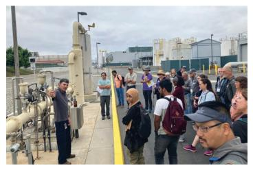
FIGURE 2, STOP # 1. OCWD HYDROLOGIST JOHN BONSANGUE SHOWING ONE OF SEVERAL INJECTION WELLS. OCWD HAS ONE OF THE LARGEST WATER INJECTION SYSTEMS IN THE U.S. USED FOR COMBATING COASTAL SALTWATER INTRUSION.
