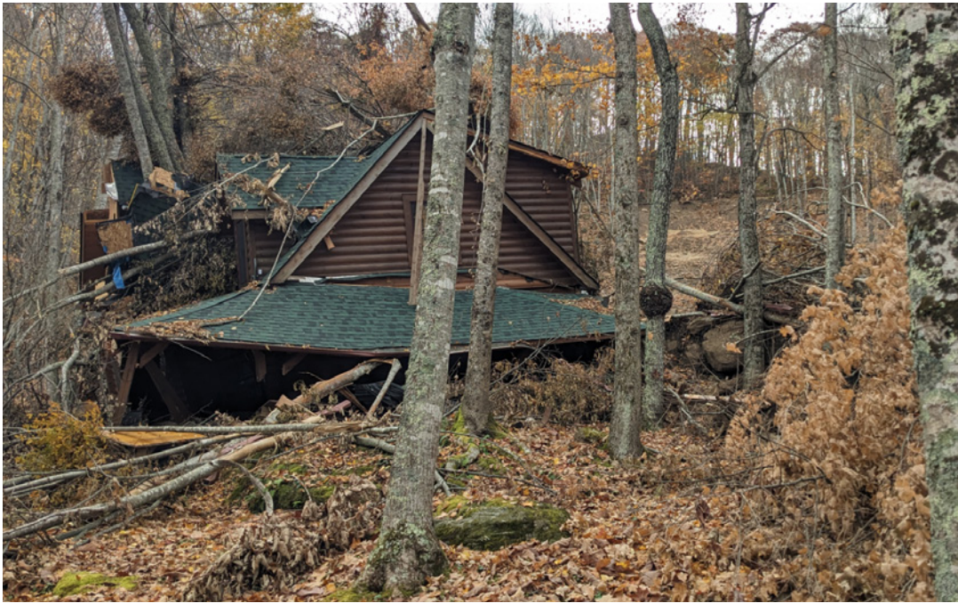
Haywood County home destroyed by road embankment failure-debris flow in background
