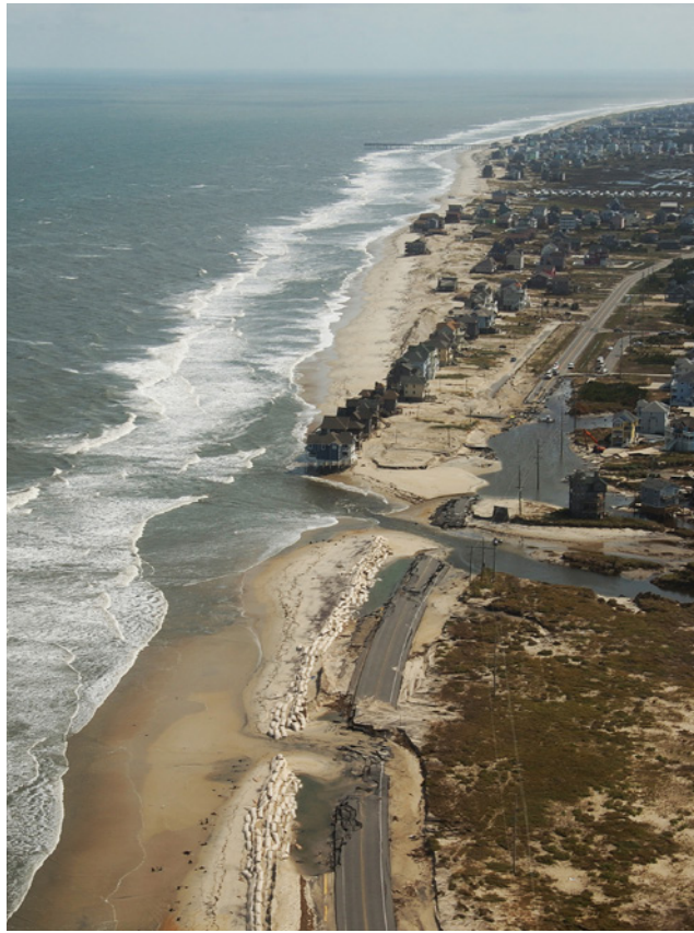
Figure 2. A breach in the coastline of Rodanthe, North Carolina, caused by Hurricane Irene in 2011. Photo by Karen Morgan, USGS.
