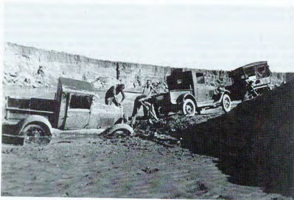
Figure 2. Crossing the Rio Puerco, flanks of Mount Taylor, New Mexico, 1930, with three 1928 Model A Ford pickup trucks, tow chains, shovels, muscle, and lots of willpower. This work was associated with Survey Bulletin 860-B (1936) and Professional Papers 189-B (1938) and 193-F (1941).
