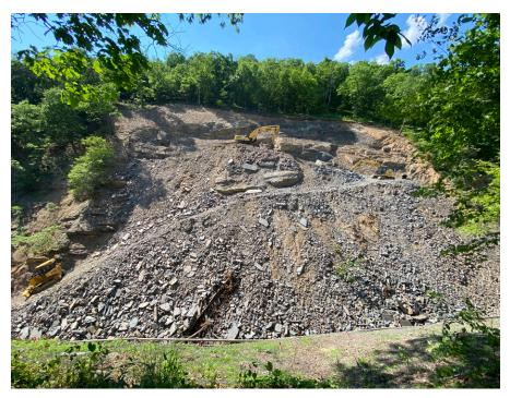
Figure 11, Establishment of switchbacks and removal of additional slope concern area and 2016 rockslide
