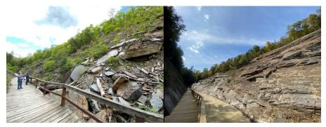
Figure 16, Paw Paw Slope Stabilization Project – As viewed looking south at the 2016 rockslide (May 2021 on left and October 2023 on right)
