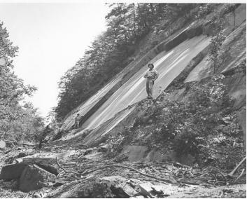
Figure 3, Rock bolting and scaling by NPS in 1950s
