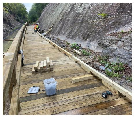
Figure 13, Boardwalk construction
