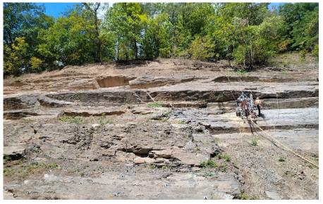
Figure 8, Rock anchor installation by rope access and wagon drill, typical
