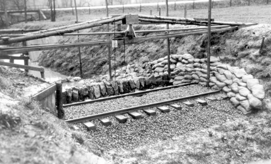
Full-size railroad embankment
