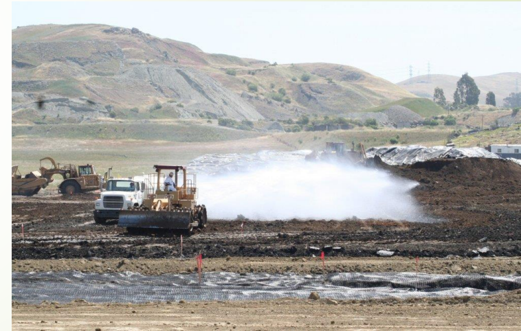
Water truck saturating soil
