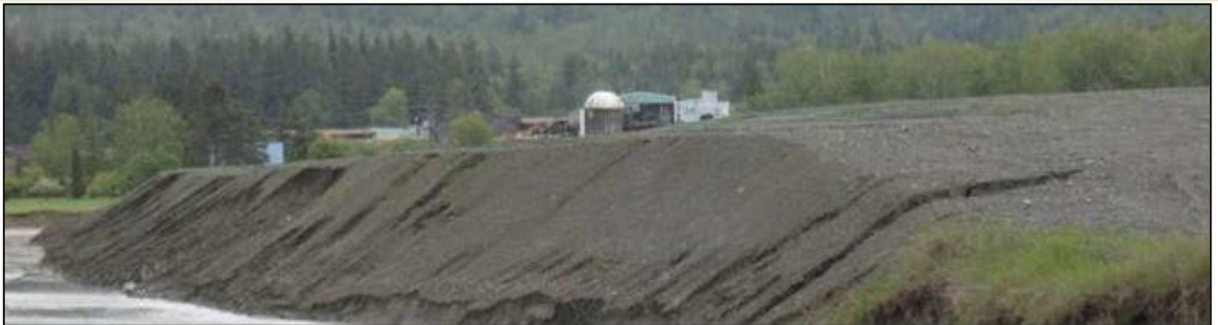
Swift Creek and dredged sediment pile
