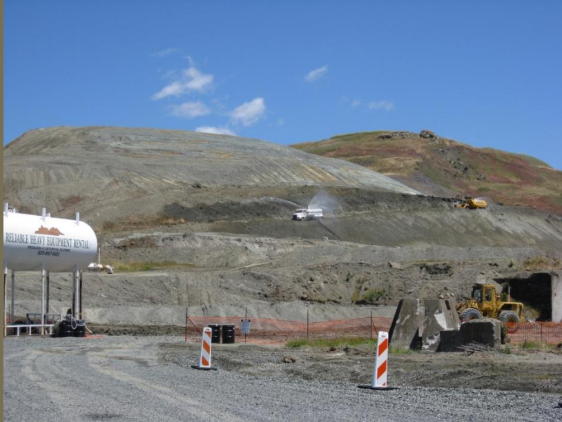
Water truck on hillside for dust control
