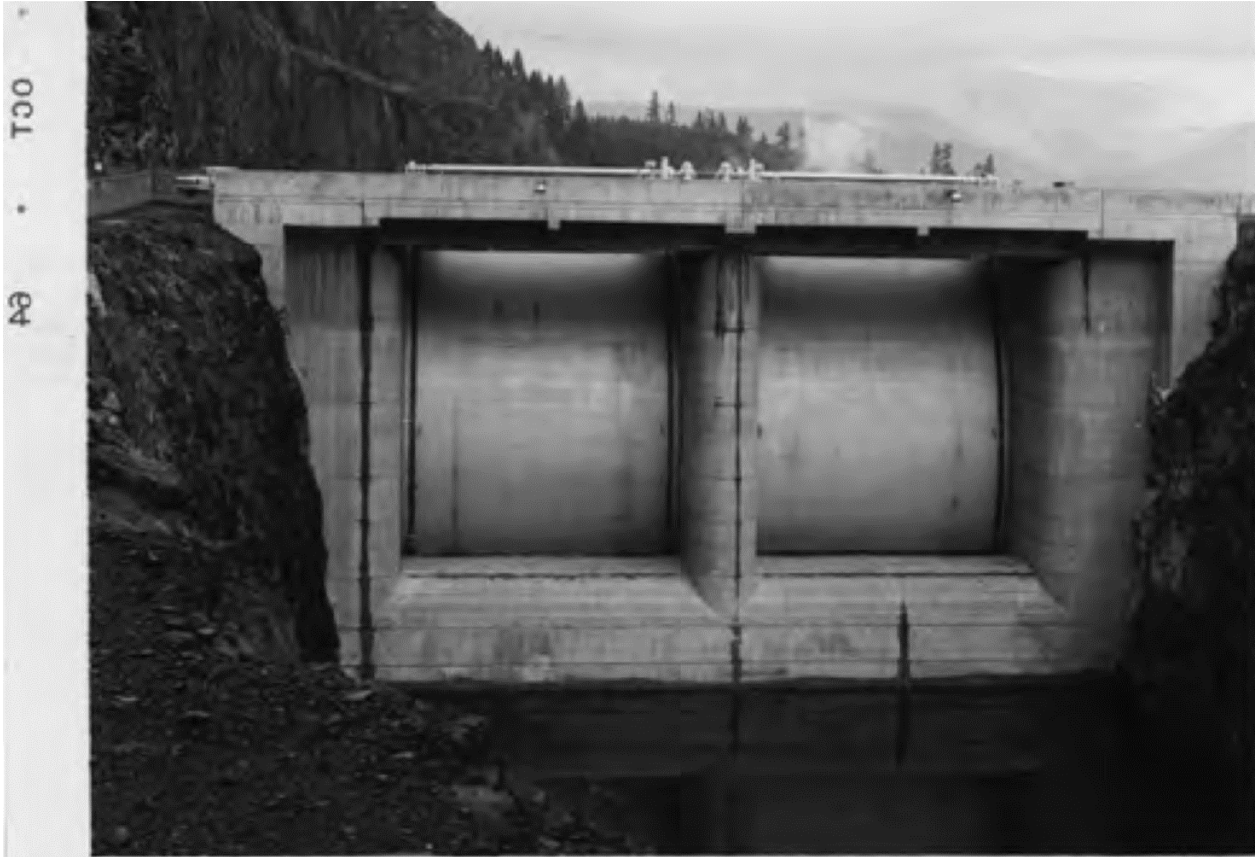
2 Tainter gates, 40-ft wide by 43.33-ft tall
