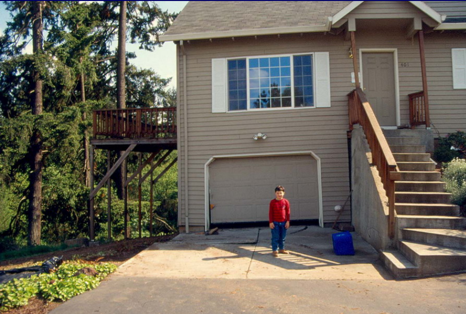
Building on the scarp
