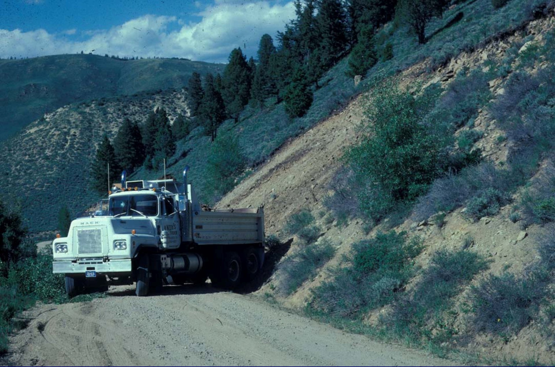
Removing landslide material from road, Sulphur Springs, Colorado
