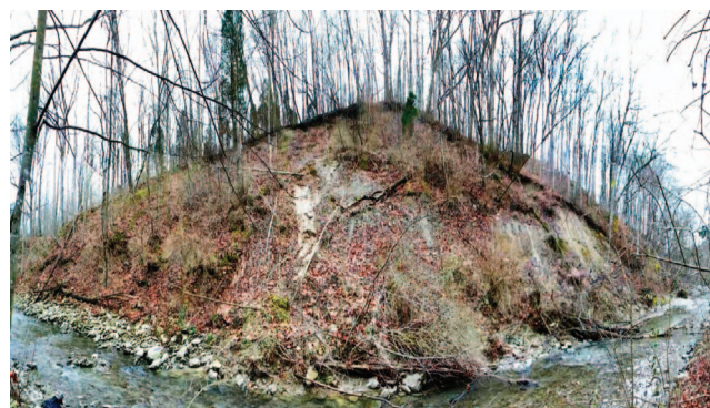
Figure 5. The Ten Mile Road landslide with well-developed head scarp. Notice the undercutting of the toe by a stream.
